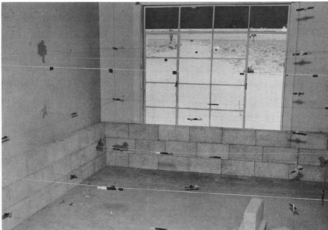
Fig. 2.30—Interior of the rambler house with 24-in.-high concrete-block wall.
